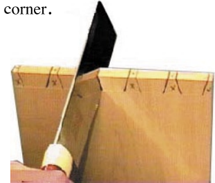
Hand-Dovetailed Joinery
