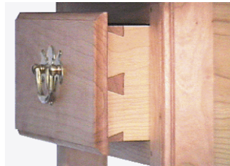
Hand-Dovetailed Joinery
